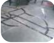
Filling the Cracks
